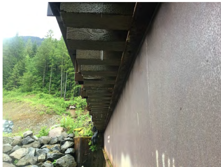
Downstream deck connection
