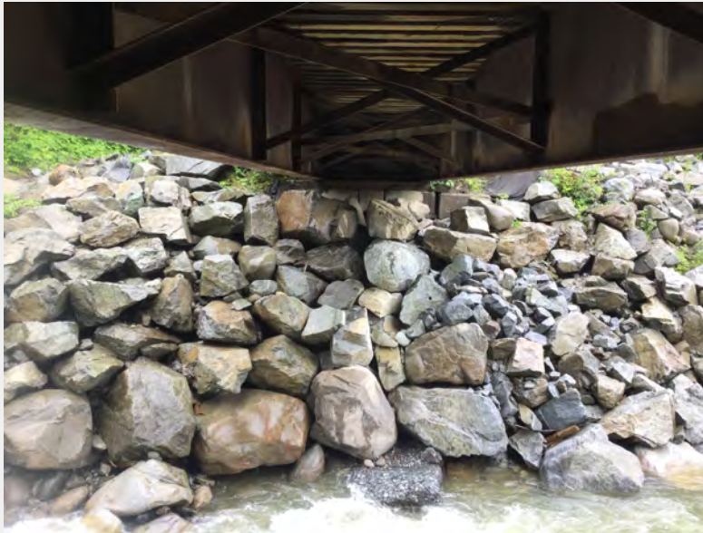
Left bank Abutment when facing downstream
