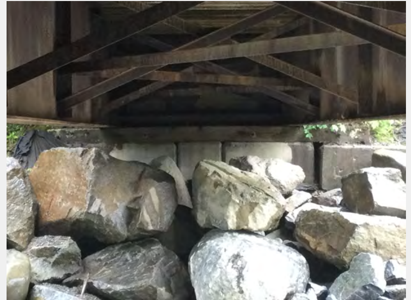
Left Bank Abutment when facing downstream
