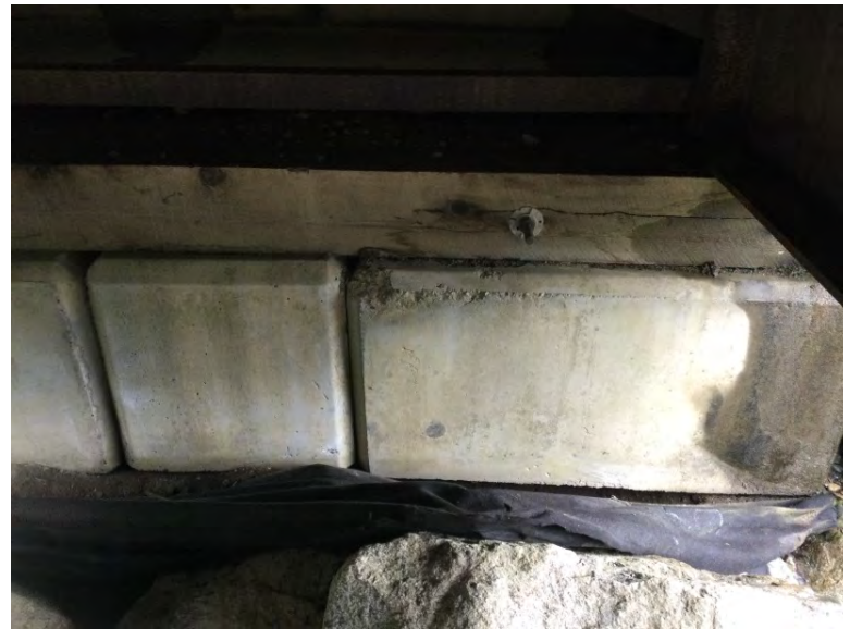
Left bank abutment
