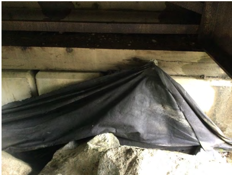
Left bank abutment
