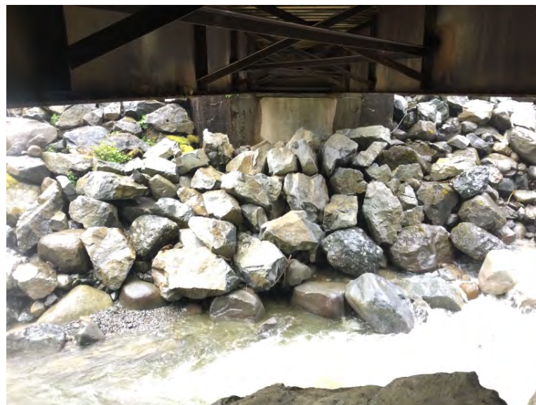
Right Bank Abutment when facing downstream
