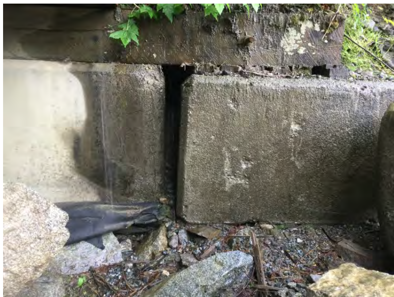
Downstream lock block left abutment
